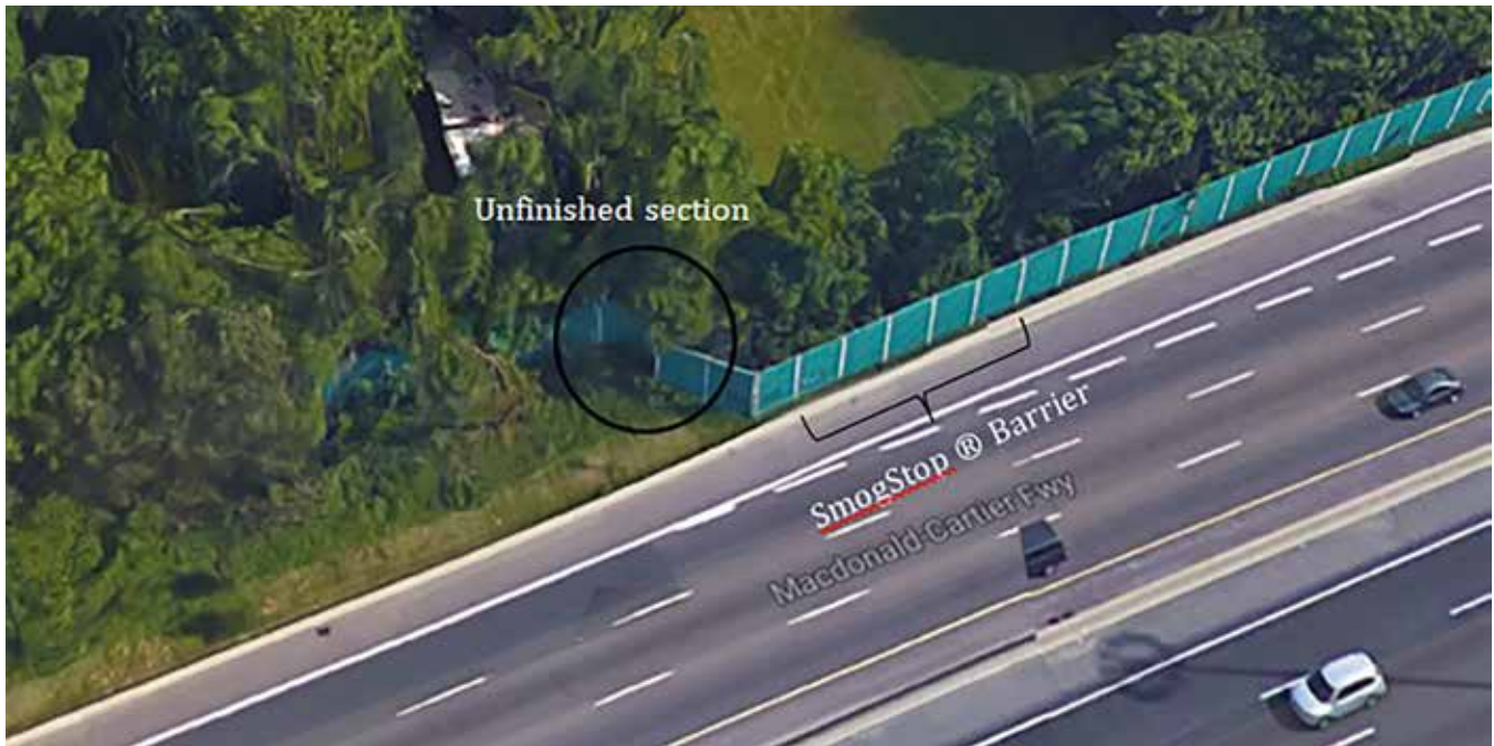
Figure 7: 3-D Google image of the field site identifying the SmogStop™ barrier location and the unfinished section (The image was taken prior to the construction of the new noise barrier, however, the opening remained in place due to underground infrastructure.)
